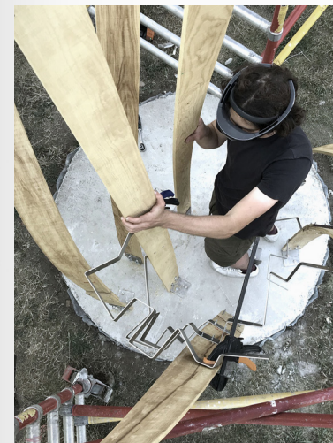
No mesurements are used in the positioning of the beam
