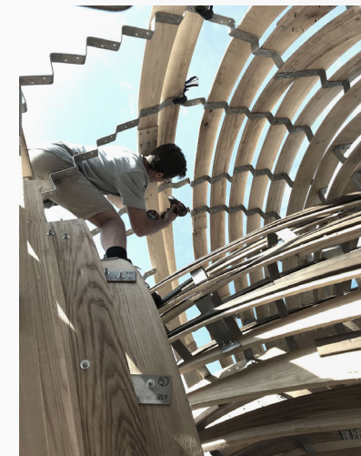
Beams and brackets are fastened with simple bolts, nuts and washers
