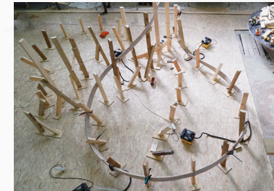
The bend structure is drying while in the form
